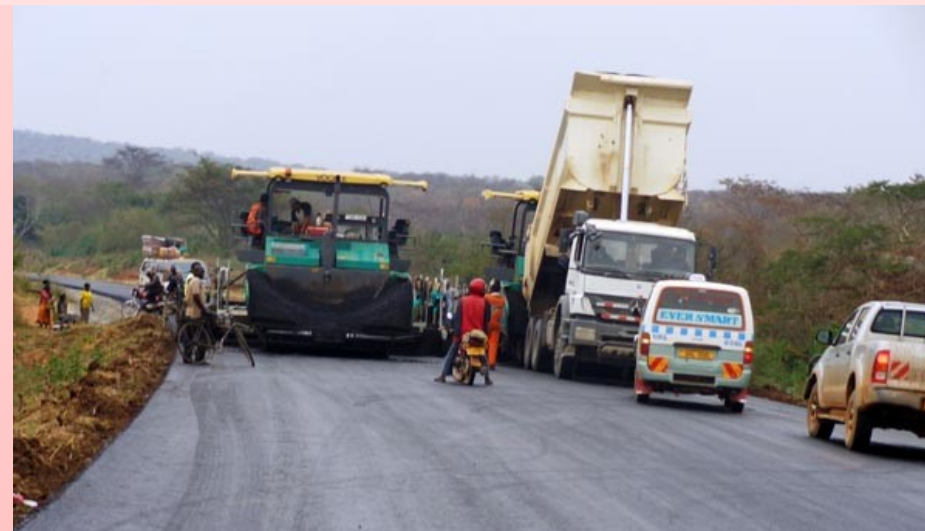
Hoima-Kaiso Tonya road being tarmacked by Kolin construction Ltd., courtesy of Daily monitor.
