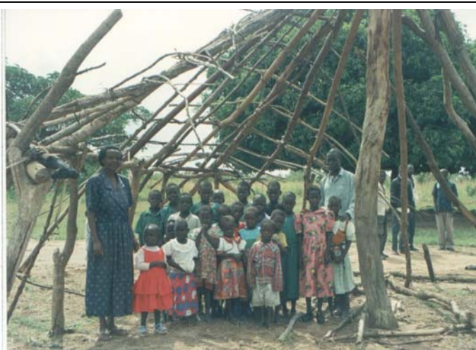
Catherine Imalingat stands with her pupils inside a classroom with a grass thatched roof blown off.
